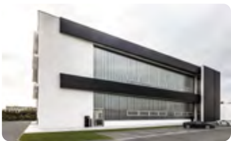
PSC & Protoshop Client: Automobili Lamborghini First multi-storey class A industrial building in Italy Year: 2013
