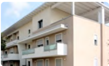
“Il Glicine” residential complex Client: Il Glicine The first multi-storey class A building built with an XLam wooden load-bearing structure in Emilia Romagna. Year: 2013
